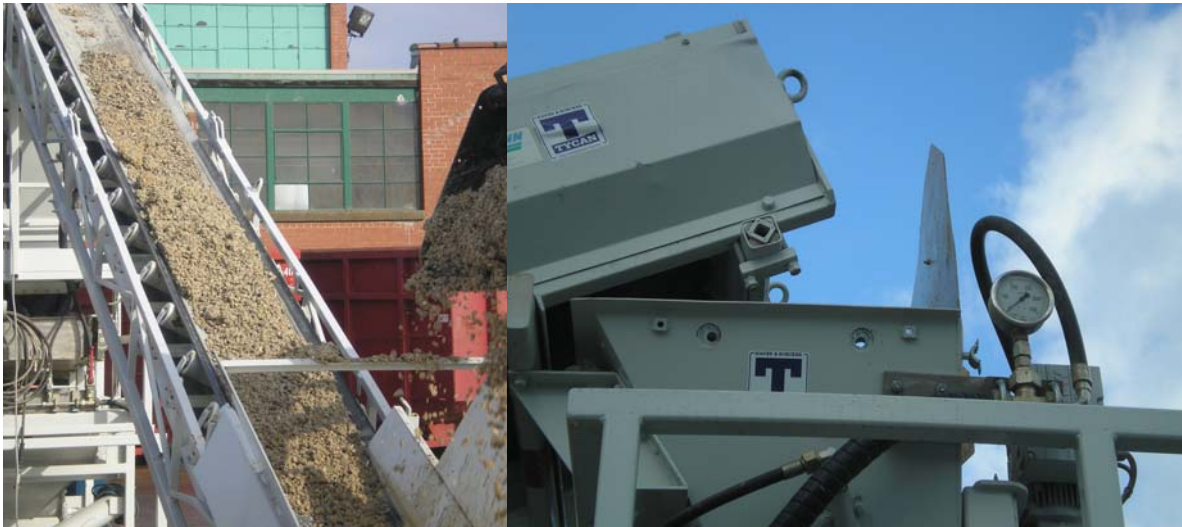
Figure 2 - Contaminated Gravel Being Transported to the Hydro-Clean Feed Hopper
